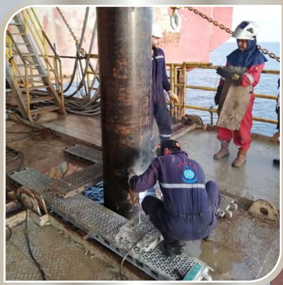
Working on Casing while Operation is Going On
