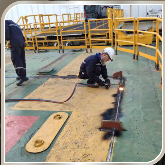
Opening Deck Hatches to remove Drilling Equipments
