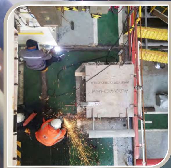
Deck Removing For Replacement Of Sewage Tank
